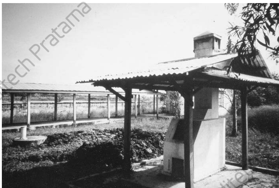
Fig. 8.3 Single-chamber incinerator
